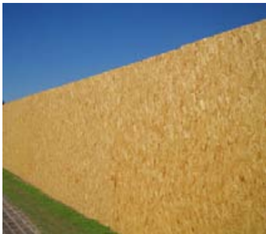
Figure 7. O.S.B. panels used as a temporary fence (photo by L. Sebastiani).
