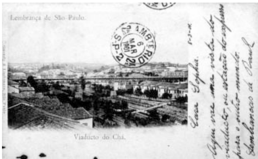
Postcard 2 (front): “Viaduto do Chá” [Tea Viaduct] (Collection Aparecido Salatini) – Message: “5-3-01. Dear Sophia. Here goes a view from the viaduct, or station of the other-world express. Greetings from Raul”
