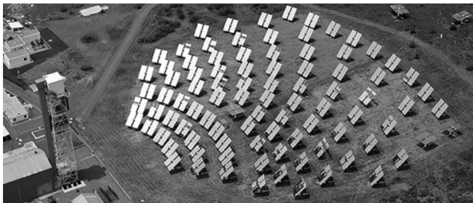
Figura 6. Central Small Solar Power Systems (SSPS).
