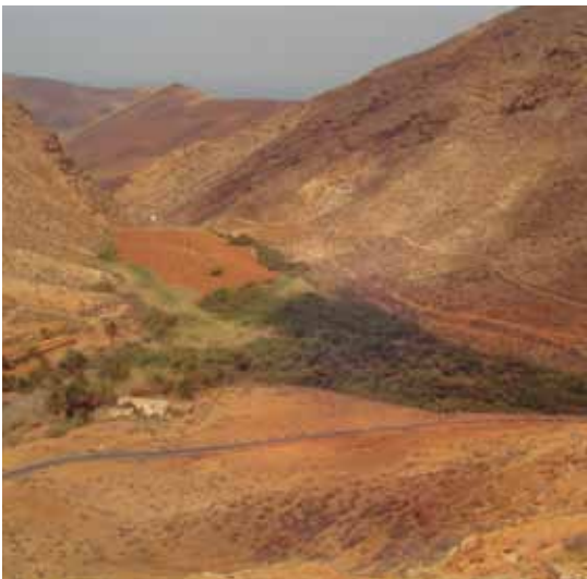
Figure 5. The La Peñita reservoir (upstream view), completely silted up. Image J. Porta.
