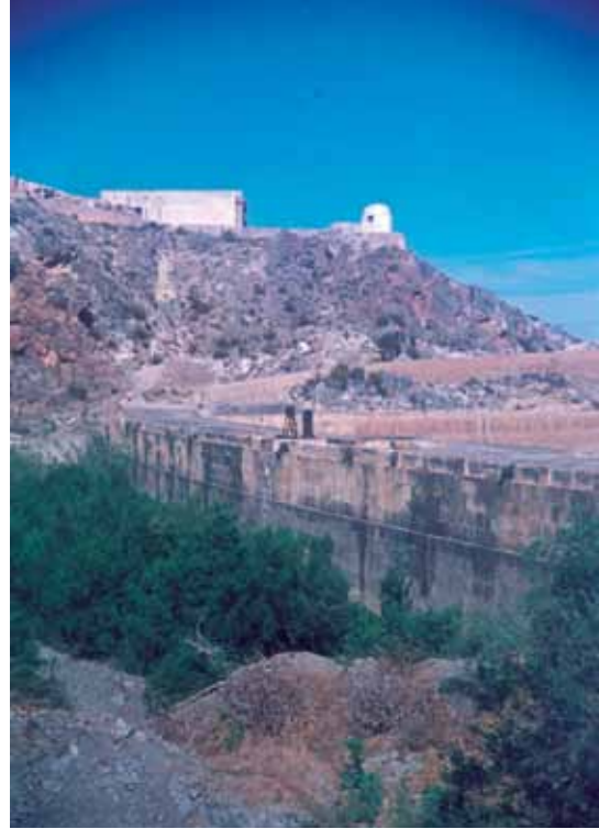
Figure 4. The Nijar reservoir (upstream view): the dam is completely silted up and has been abandoned since the beginning of the 20 th century. Image J. Porta.
