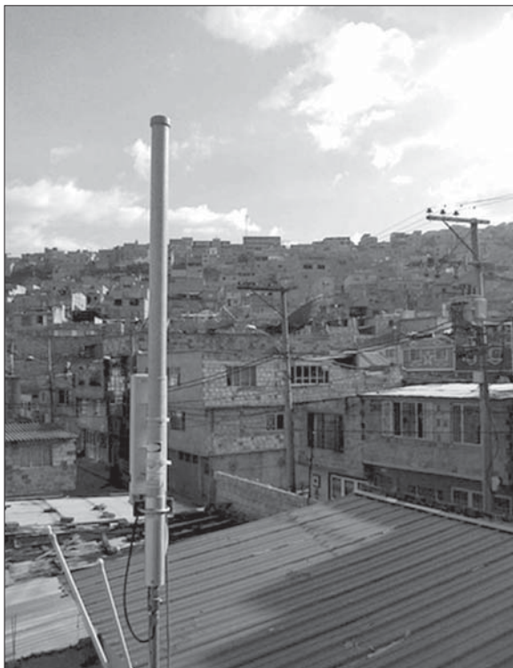
Figure 5. A Bolivar wireless implemented node
