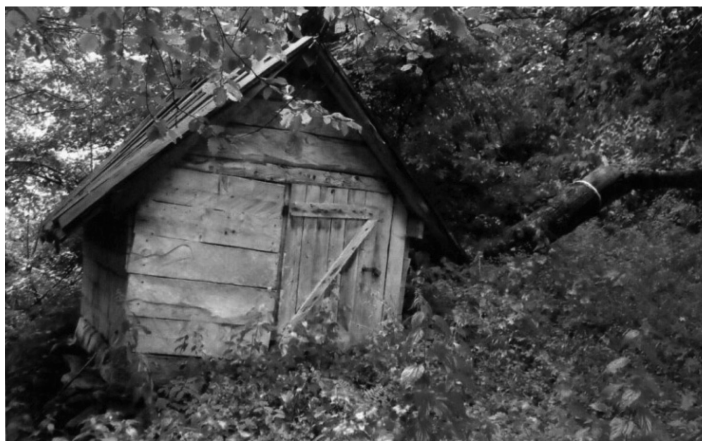
FIGURE 7. Watermill “Božovića” - resist the ravages of time
