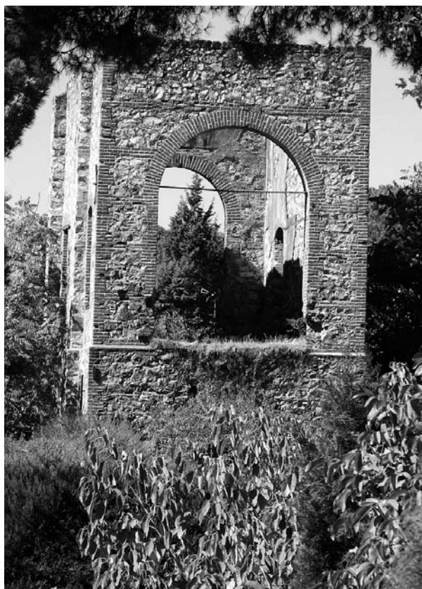
Figure 9. The San Rafael Shaft engine house that once contained the Hathorn Davey engine. The photograph was taken in 2004.
