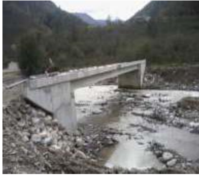
Picture 6. A 21st century bridge during which is under construction.
