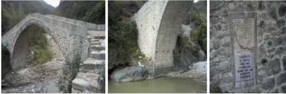
Picture 1. 13th century bridge (restored).
