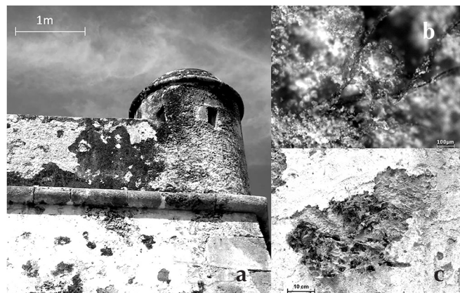
FIGURE 4. Biological activity at the San Carlos Bastion: (a) General view of biological colonization formed over east wall; (b) Mortar disintegration induced by hyphae penetration; (c) Mortar damage —consequence of biological activity— (Photograph: Javier Reyes, 2010).
