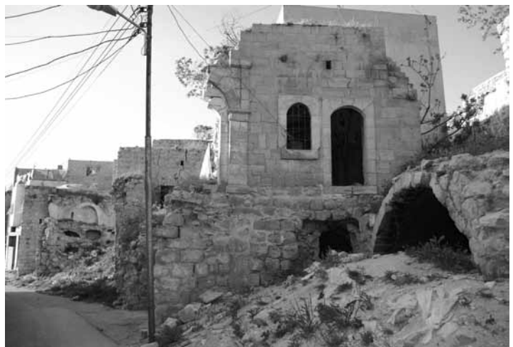
Figure 3. Hebron: Salaymeh Destroyed Heritage. Photo BSP
