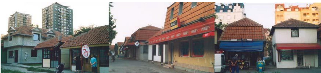
Kiosk architecture: private commerce and individual housing. Photo: 2003
