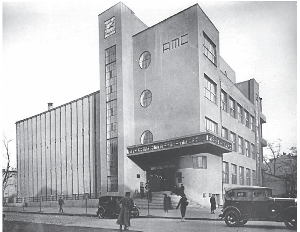
[Fig. 6] Automatic Telephone System building, 1930-1931, arch. P. I. Frolov. Source: prof. A. Bouryak's personal archives.
