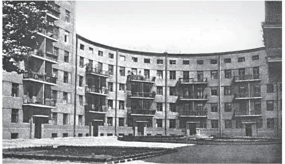
[Fig. 14] Kommunar (Communard) residential house, 1929-1932, arch. A. V. Linetskyj and V. I. Bogomolov. Source: prof. A. Bouryak's personal archives.
