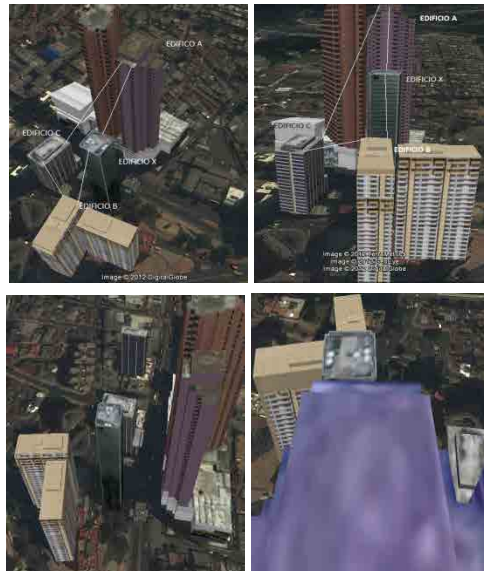
FIG. 2. Different views of the three buildings taken in Google Earth.
