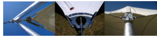
Figure 10. The cable is attached to the mast and fabrics (Mahmoud et al 2013)
