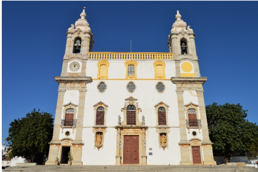
Figure 17: South facade of the Church of the Carmo of Faro.
