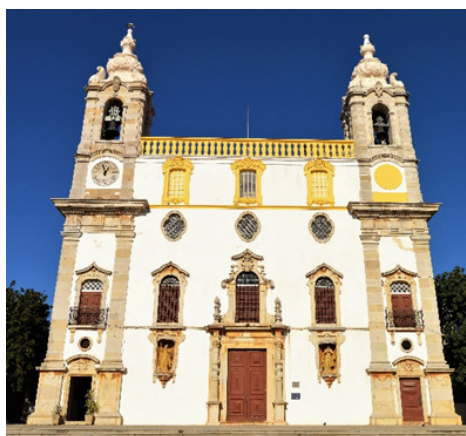
Figure 15: Main façade from the church of the Carmo of Faro to the south.
