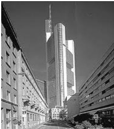
Figure 8. The Commerzbank office tower
