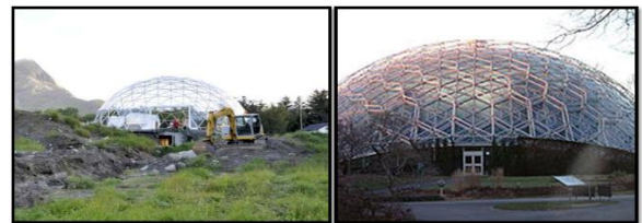
Figure 4: Two-layer geodesic dome (right, Missouri Climatological Botanical Garden) and a geodesic dome of a solar layer (left, corn cobwebs of Norway houses)
