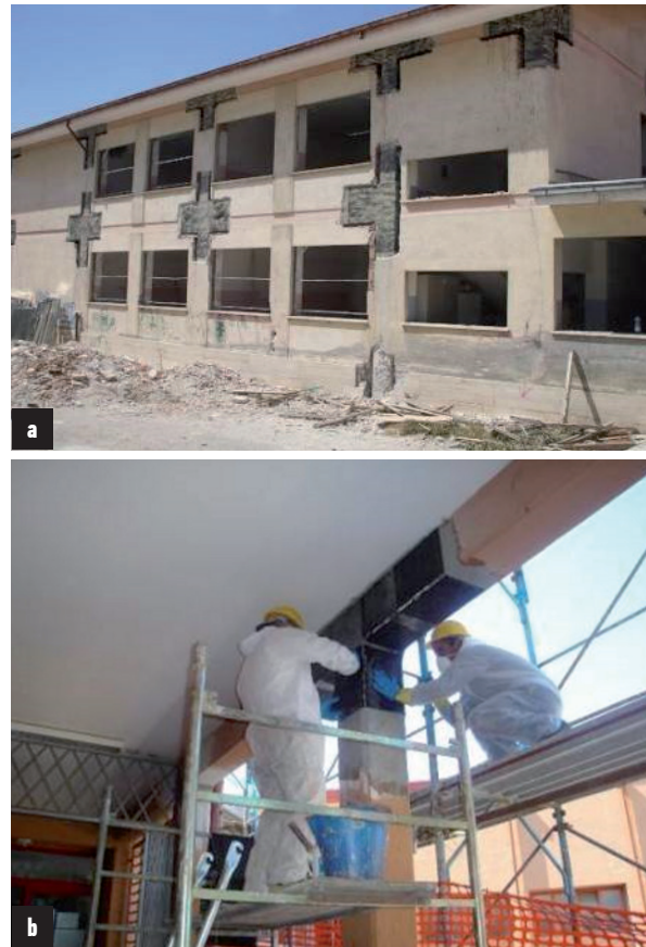
Figure 3. Prep work and strengthening of external joints.
