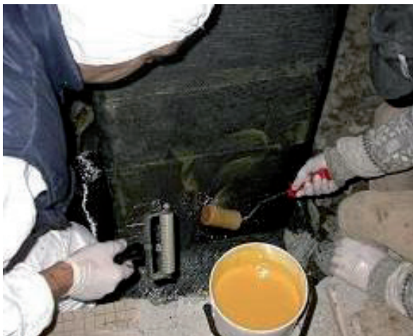
Figure 5. Strengthening of column by full CFRP wrap.
