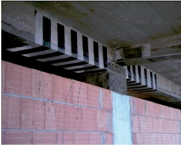
Figure 4. U-shaped CFRP wraps.
