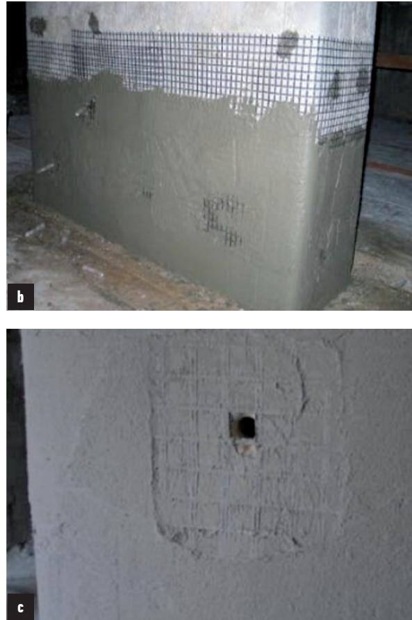
Figure 10. Application of mortar followed by carbon fabric and spikes.
