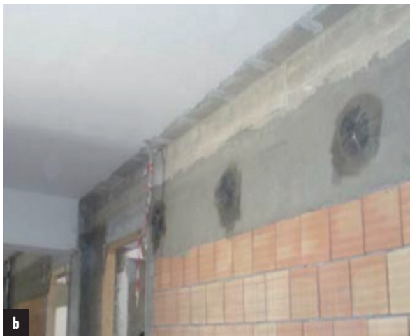
Figure 7. Partition anti-overturning repair with FRCM and SRP spikes.
