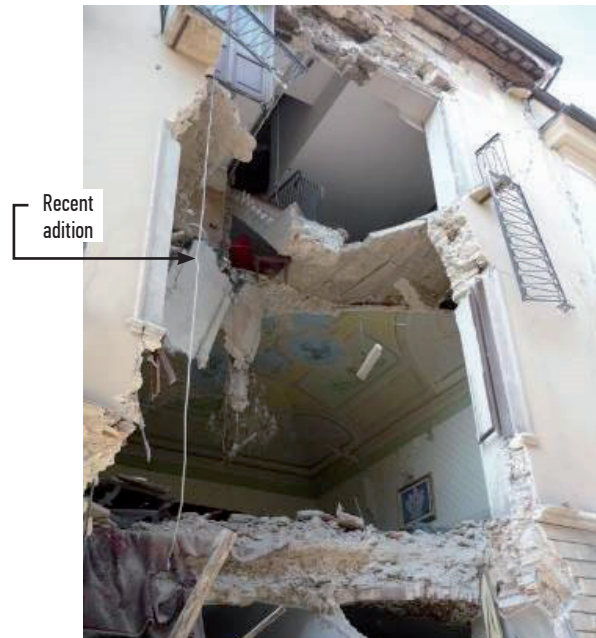
Figure 8. Damage resulting from insertion of concrete stair.
