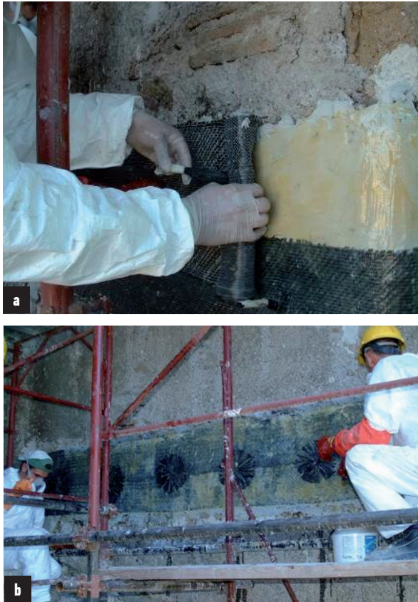
Figure 9. Wrapping with CFRP plies anchored with CFRP spikes.
