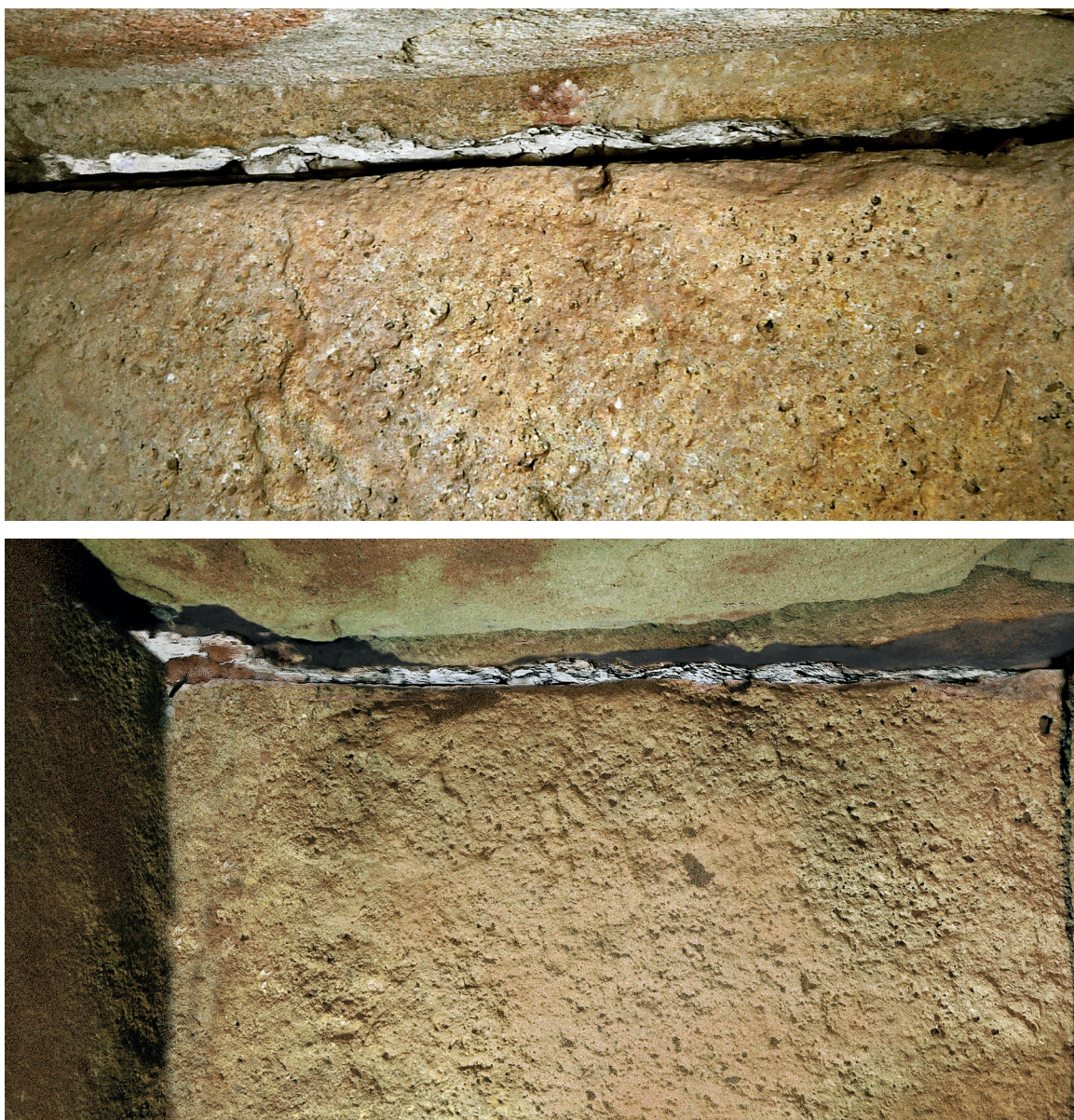
Fig. 9. Upper section of the entrance door from Viera's chamber. It can be appreciated the cutback of the support as well as the lime covering of the chamber. Photography by R. de Balbín.
