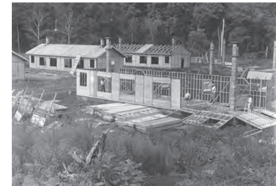
Figure 4. Maekawa Kunio. PREMOS, Construction Process. Provided by, Mayekawa Associates, Architects & Engineers.
