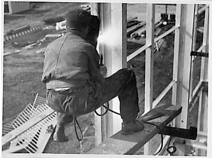
Welder at work - continues welding rebar stair components below.
