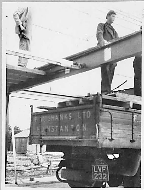
Flow slab fixing Shanks' men.
