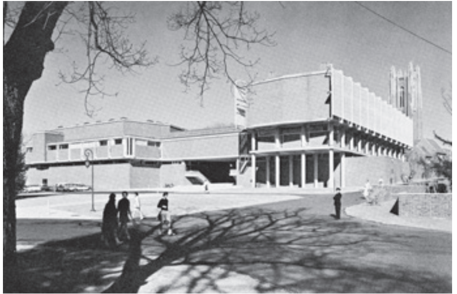
[Fig. 9] Paul Rudolph. Jewett Art Center en Wellesley, Massachusetts, 1955-1958. Fuente: Timothy M. Rohan, The Architecture of Paul Rudolph (Yale University Press: 2014), 40.
