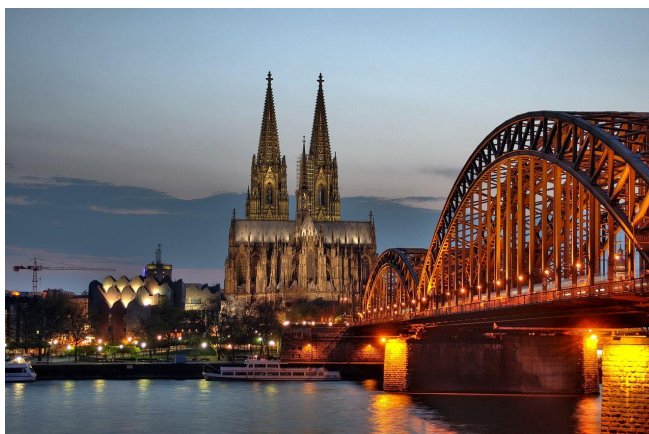
The Cologne Cathedral with the Hohenzollern Bridge
