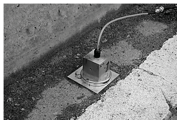
Figure 10. Sensor on the bridge. From: [13].
