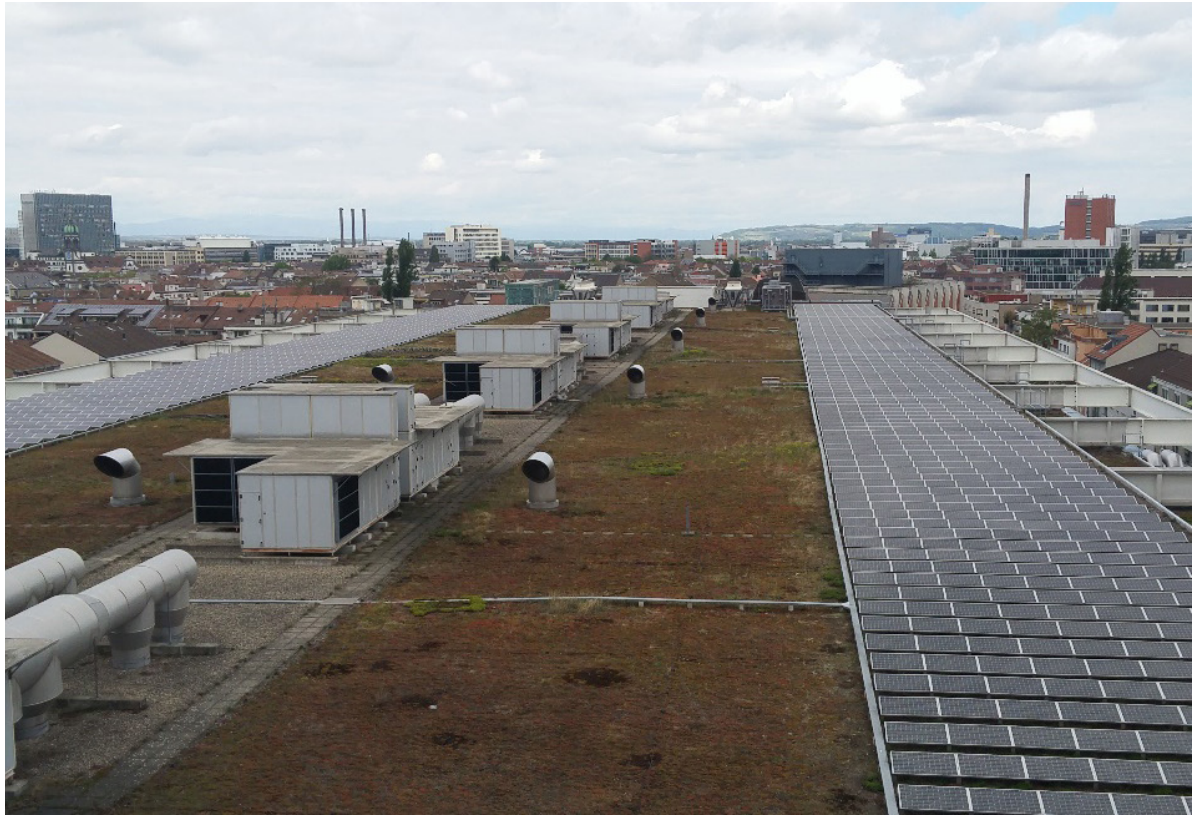
[Fig. 5]. Basel, Convention Center roof, Herzog / de Meuron, 2013. Source: the author. Fuente: el autor.
