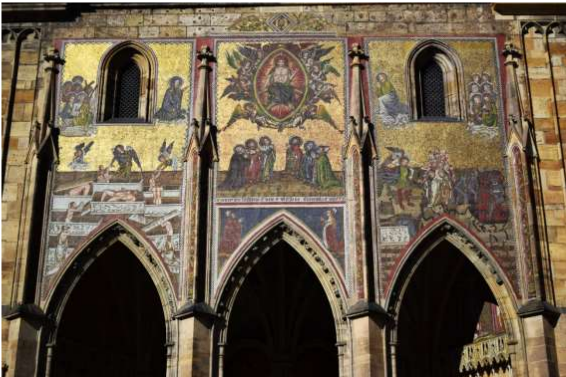
Fig. 7: South façade of St. Vitus Cathedral. Prague. (GumielCampos ©)
