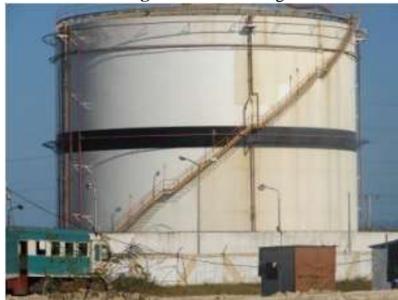
Figure 1: Fuel storage tank.
