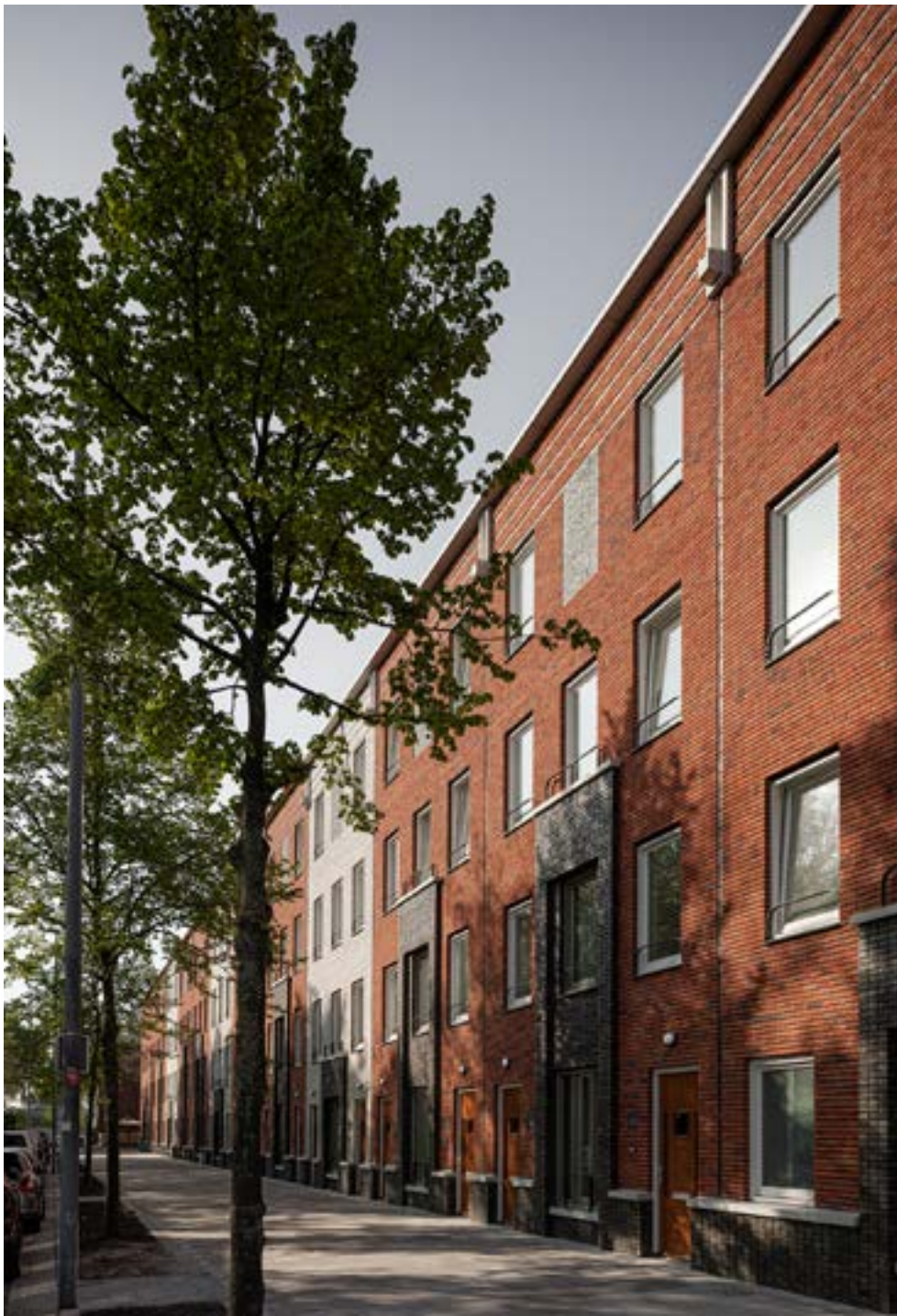
Façade along Persoonshaven (Sebastian van Damme)
