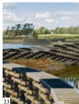
Figure 24 Weaving pattern of river walls constructed with timber
