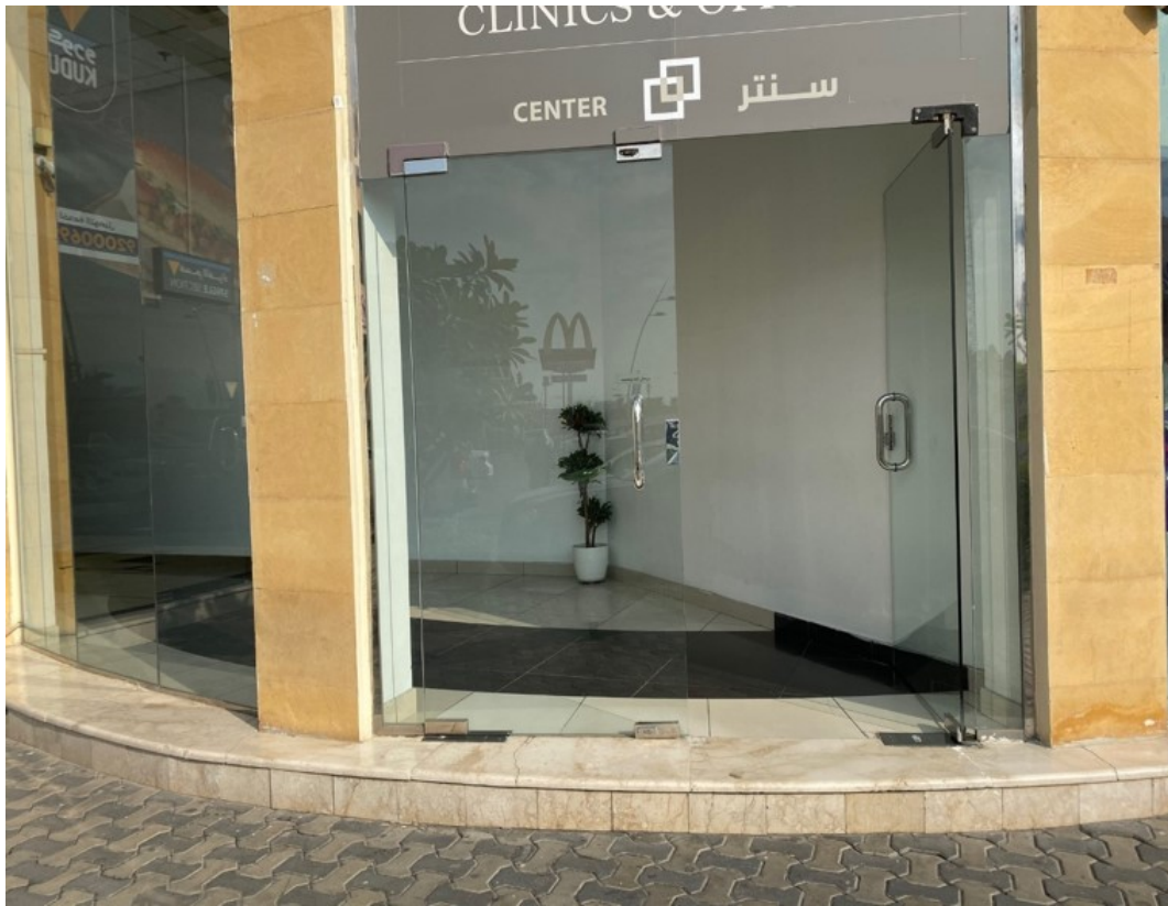
Figure 4. Entrance to office and clinic building. Source: photo- author archives.
