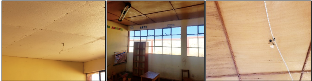
Figure 7. Existing false ceiling: 4mm plywood sheets, fixed to the lower part of the wooden scissors in 1.22m x 1.22m panels, joined with wooden flashing, with varnish paint finish.
