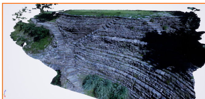
Figure 8. Photogrammetric recreation of the east retaining wall. Photos by A. Burbano, processed by Z. Meyer, 2020.
