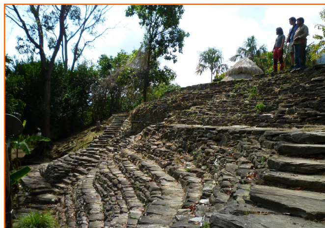
Figure 4b. Retaining wall and stairs on the east side of main terraces in CA. Photo by E. Mazuera
