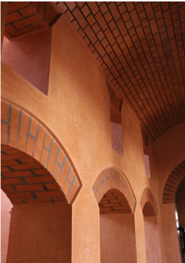
Interior details with glazed brickwork and tadelakt finishes
