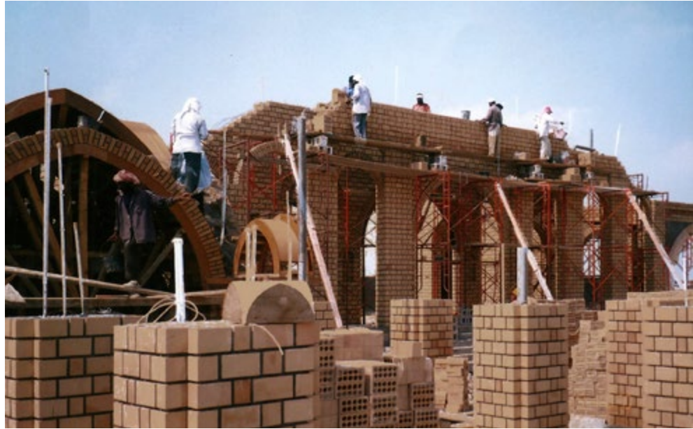
Construction of Dar Al Qasir, Manama, Bahrain, 1995
