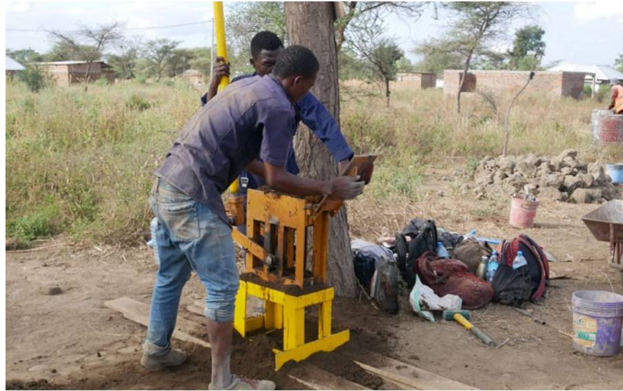
Figure 15: Two skilled workers producing compressed stabilized earth blocks in Maji Moto
