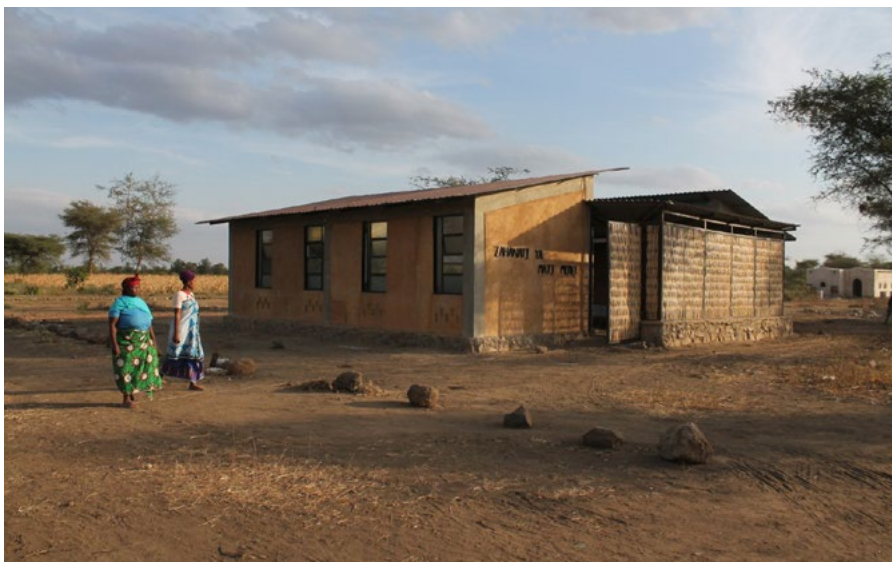
Figure 14: Health center built with compressed stabilized earth blocks in Maji Moto
