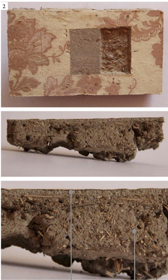
Enlucido : 4 mm of soil and sand plaster Enfoscado plaster: 30mm of soil and fiber
