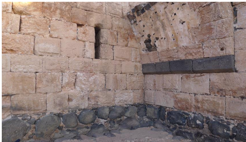
Fig. 6 – Vault inserted in the wall.
