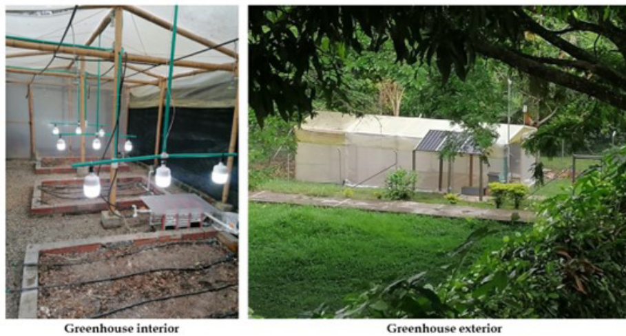
Figure 5. Physical internal and external structure of the greenhouse.
