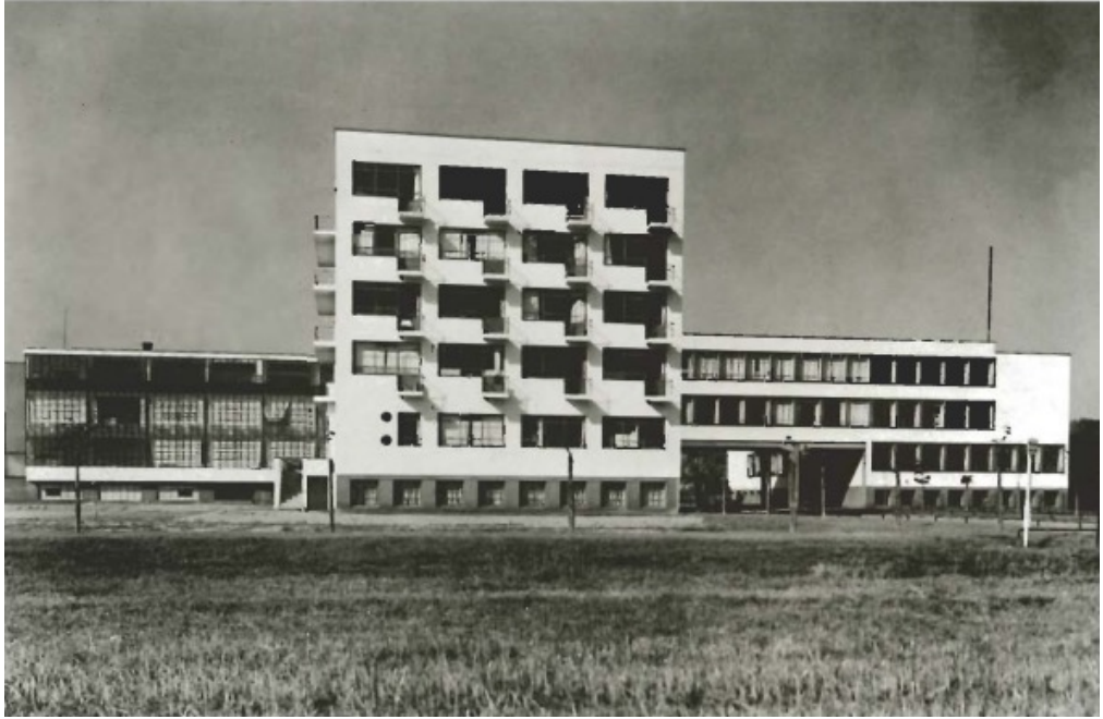
Figure 6: East view of the Prellerhaus (Dessau, 1926-1927)
