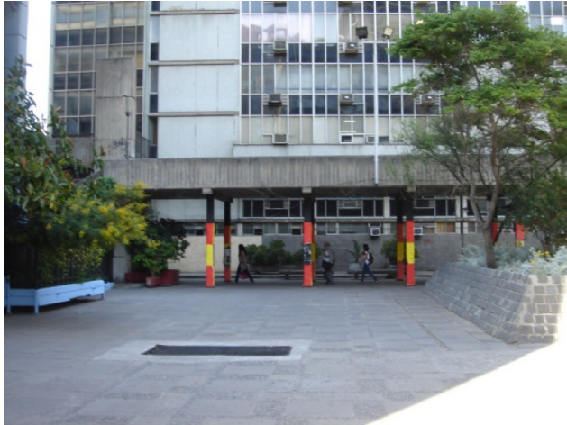
Figure 5. Underground Station at San Borja Source: Own elaboration.
