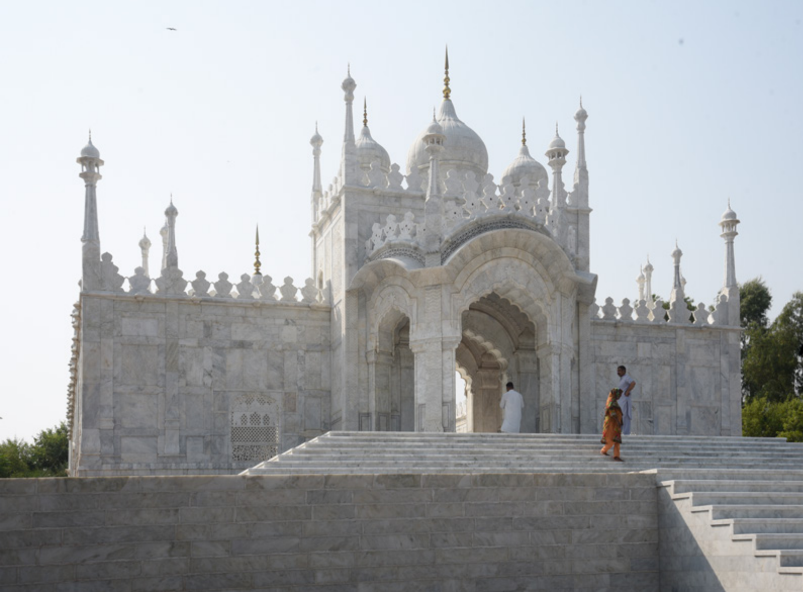
Main entrance | Entrada principal | Entrada principal (Raza Kazim)
