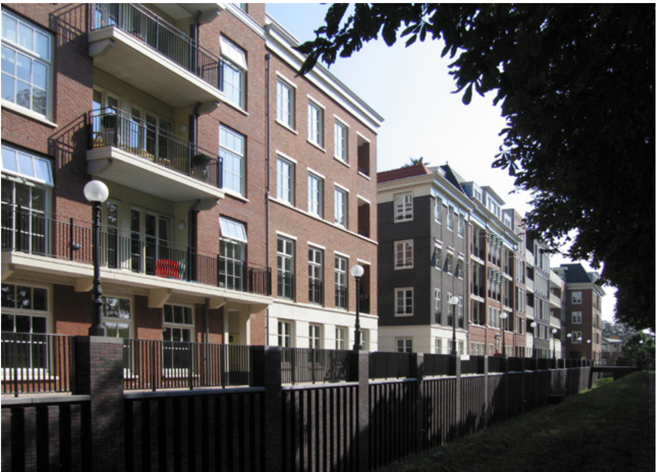
Facade balconies | Balcones de fachada | Varandas nas fachadas
