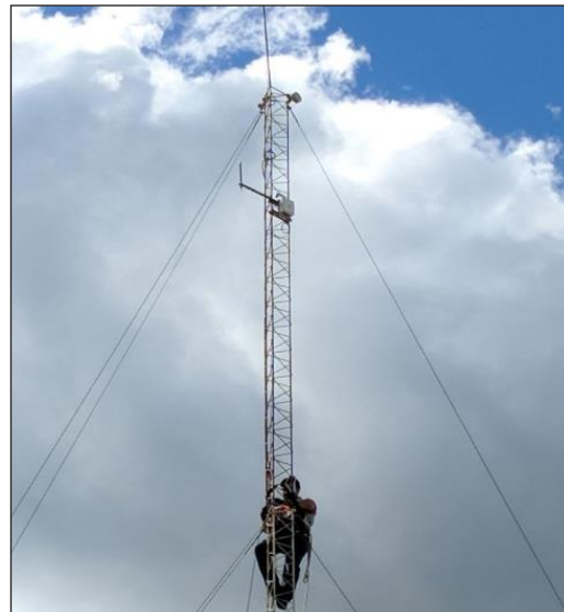
Figure 3: Deployment of a gateway at the Biochemistry building, FCEQyN.
