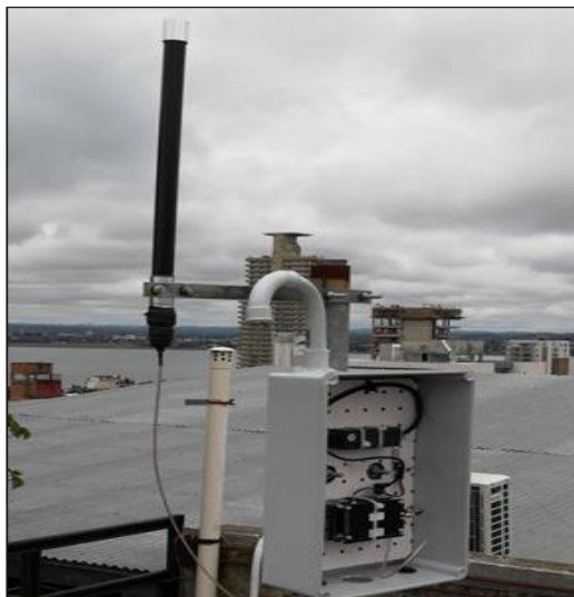
Figure 2: Gateway installed at main building of FCEQyN.
