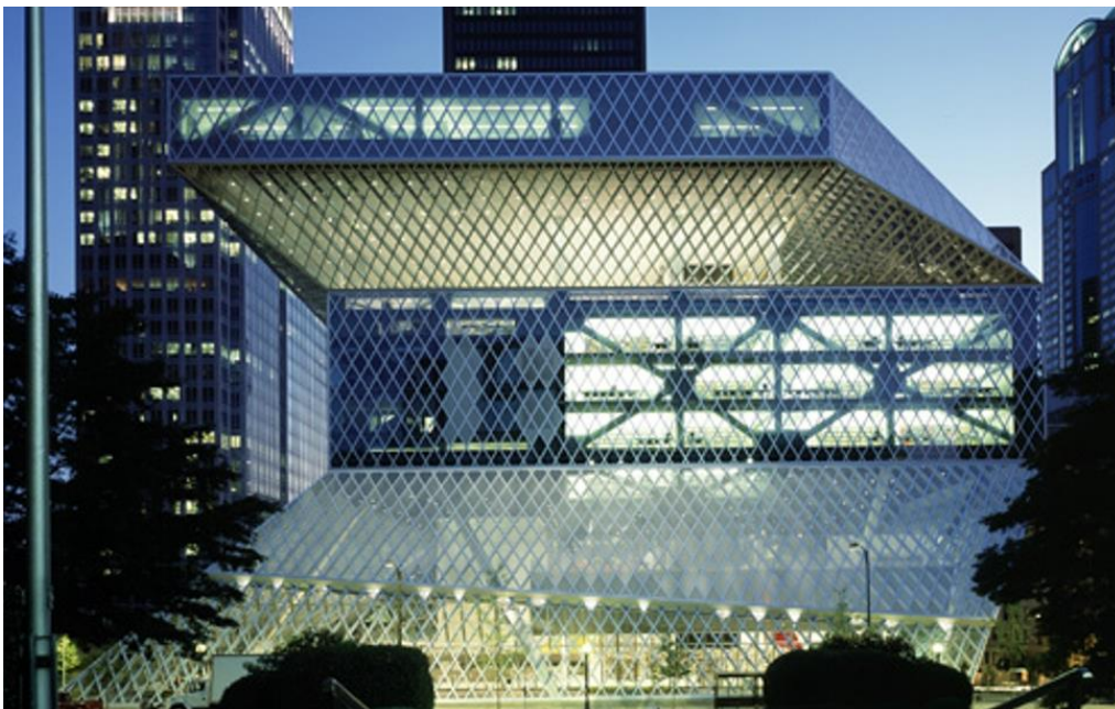
Fig. 2: Exterior Image, Seattle Library (Source: OMA)
