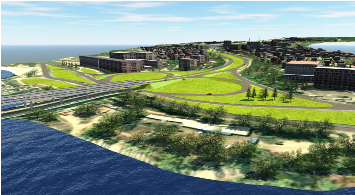
Figure 13. BIM-model of the transport interchange at the construction site of the Northern Bypass in Dnipro city.
