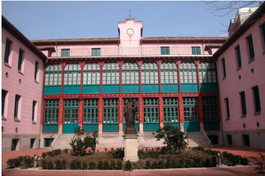
Figure 1. Emilia Checa's rehabilitation and restoration of the Homeopathic Institute and Hospital of San José, 2007
