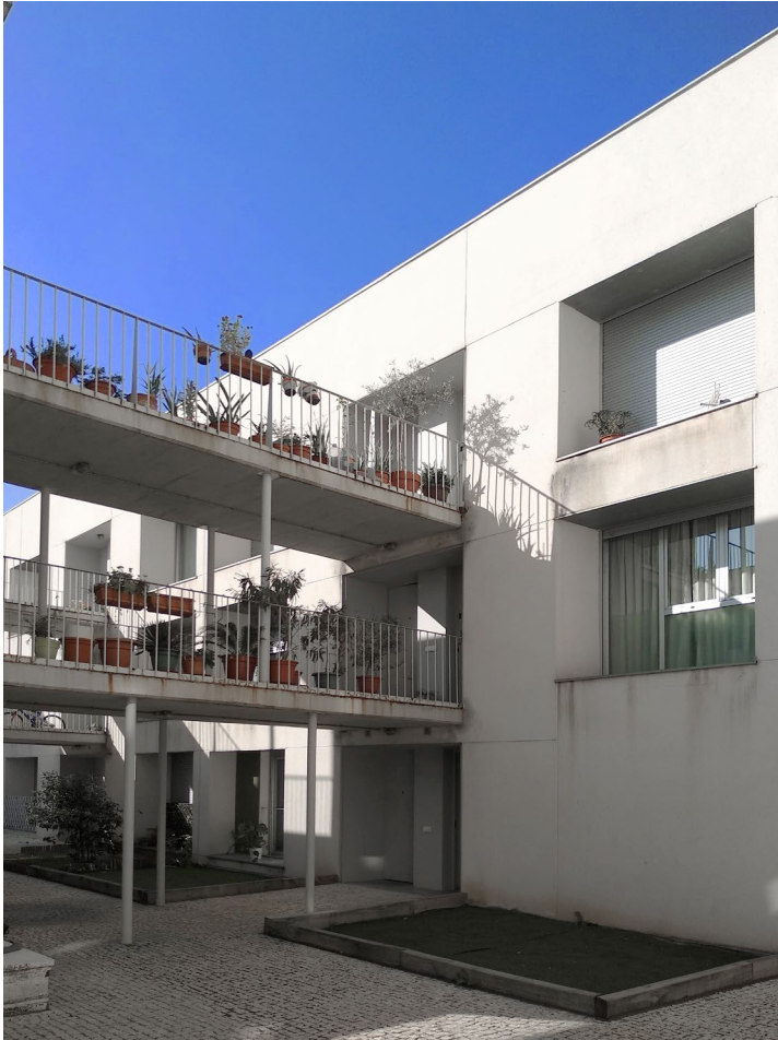
Figure 14. 122-unit social housing project (Mónica Alberola and Consuelo Martorell). Common spaces
