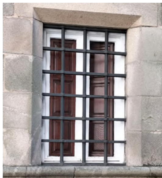
Figure 3. View of the window from San Francisco Street
