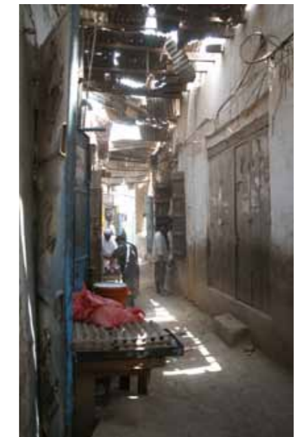
Zabid suq, Yemen: the market area of Zabid is the centrepiece of the historic town, but has lost much of its activity to a new market outside the historic town.
