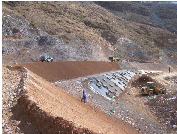
Figure 3. Landfill restoration in La Gomera (Canary Islands, Spain)
