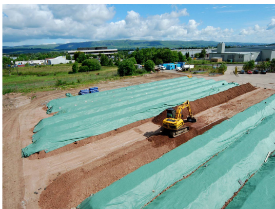
Figure 2. Bioremediation of contaminated soil (Source: http://www.tipner.co.uk ).
