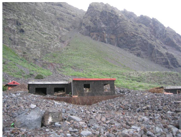
Figure 7. Debris flow deposit destroys houses in El Hierro, Canary Islands, Spain
