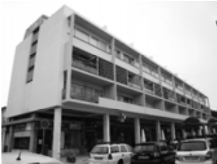
Figure 5: D. Afonso V Building, West façade.
